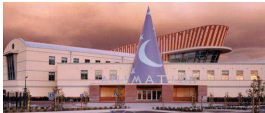
Figura 03 - Fachada Frontal do Feature Animation Building
