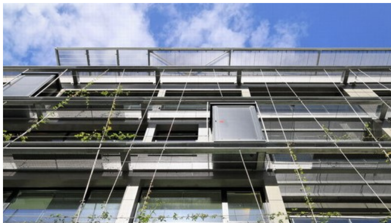
Figura 11 - Senior's Residence + Nursery - Elementos da Fachada
