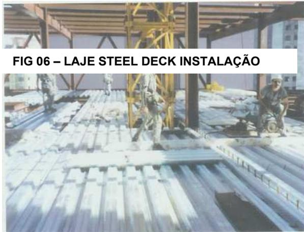
**FIG 05 – LAJE STEEL DECK**
