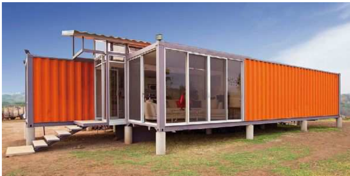
Figura 56 – Casa Containers of Hope
