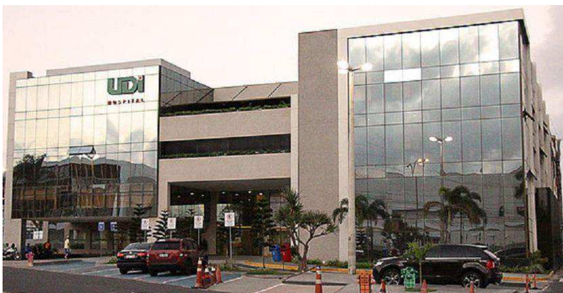
FIGURA 12: Vista frontal do Hospital UDI
